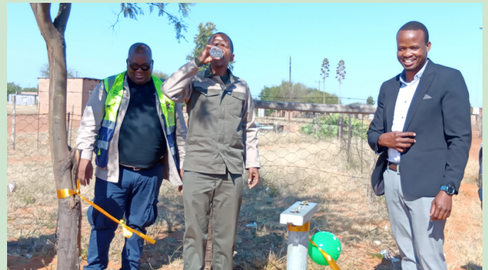
Executive Mayor, Cllr. M Maje confirming water was running from a newly installed tap by having a sip of water
