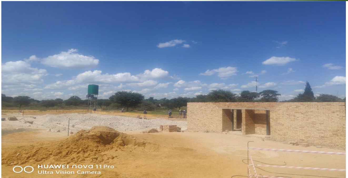
Piet Plessis Sports Facility Dressing Rooms under construction
